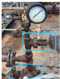
Figure 1. Valve isolating the pressure gauge.
